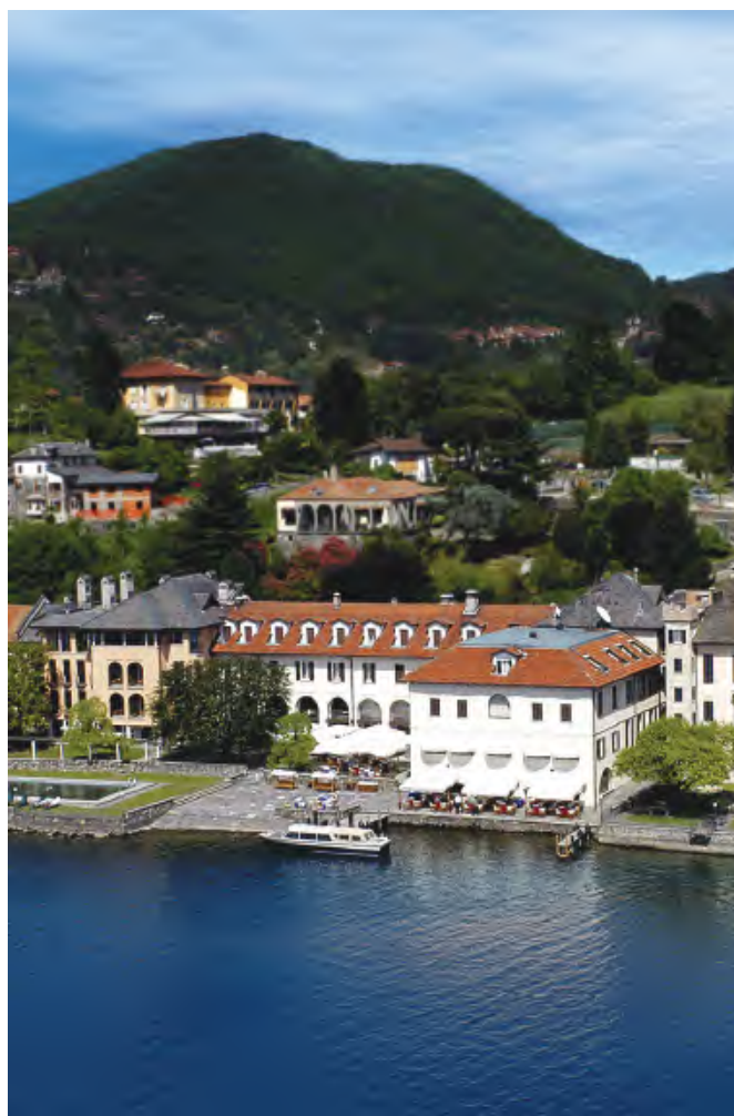
Aerial view of the San Rocco
