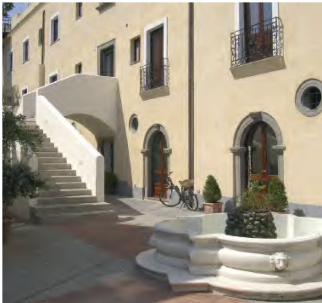
Hotel Villa Meligunis, the entrance courtyard
