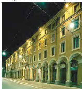
Exterior view of Grand Hotel Majestic "Già Baglioni"
